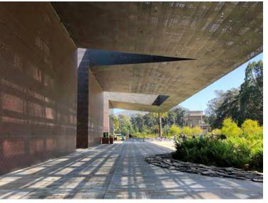
We wanted a deep dive into the exploitation of metal's inherent tendencies, and to see, up close, how the material was utilized in an extradorinary way. The digital design process for the project developed and managed 218,000 sf of embossed/perforated copper panels and nine different levels of surface texture.
