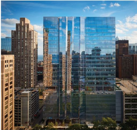
ADJACENT BUILDING | LOOKING SOUTH
