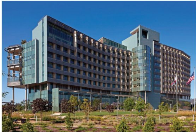
Back of the building
