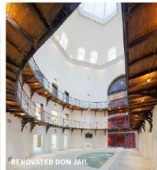
RENOVATED DON JAIL
